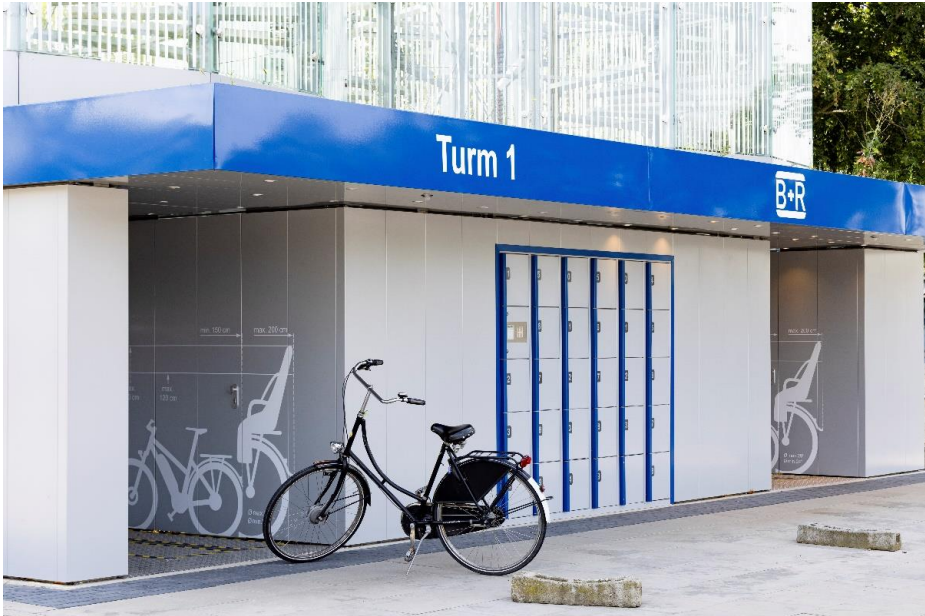
Fig 59. Closer view of the two entrances to the cycle tower. The lockers are also visible here (Copyright: Region Hannover, Terzka).
