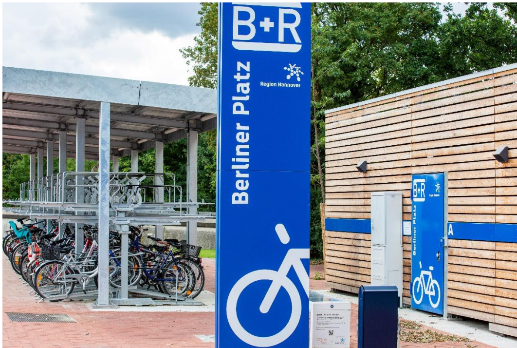
Fig 62. View from the other side of the B+R station in Langenhagen (Copyright: Region Hannover).
